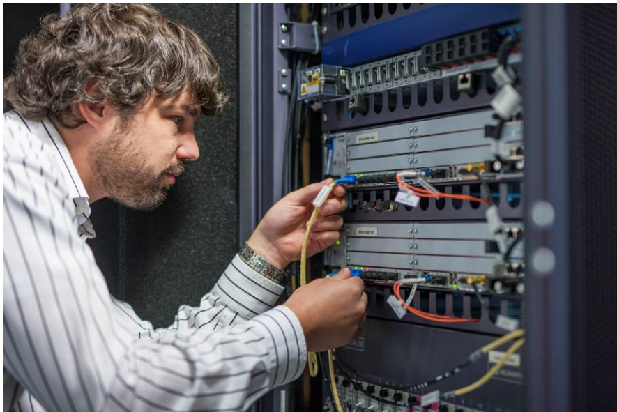
The centre's own LTE network infrastructure
