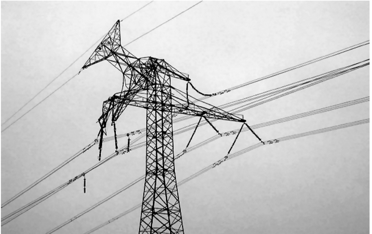
Fig. 1: Damaged Tower
